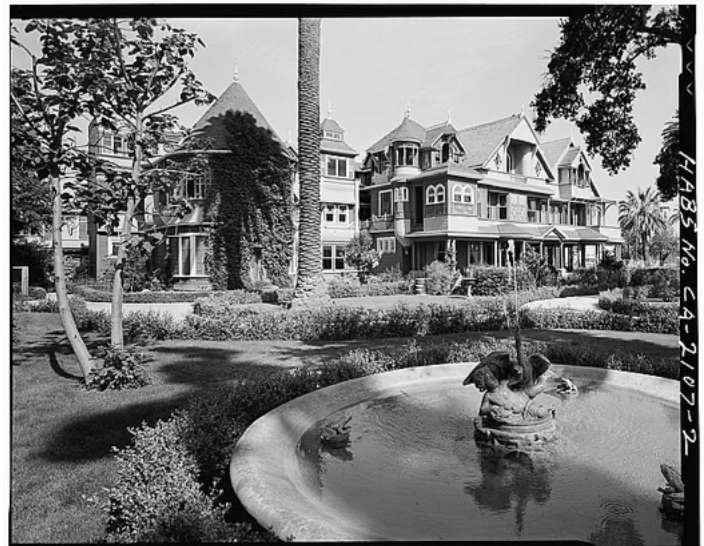
Winchester House, photographed by Jane Lidz for the Historic American Buildings Survey, circa 1933. Courtesy of the Library of Congress.
